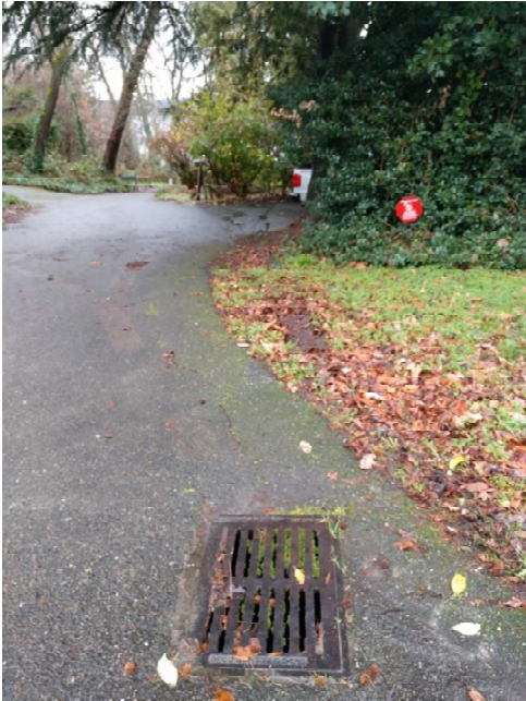
Photo S12 – Facing west in front of the entrance to Garfield Landing approximately 35 feet west of Photo S11. Runoff is conveyed west toward Lake Washington.
