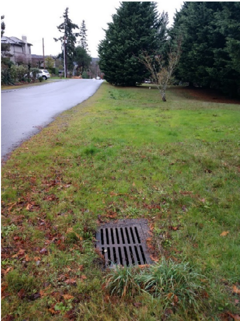
Photo S1 – Facing west along the north side of SE 30 th St. Onsite runoff sheet flows in the southwestern direction to the catch basin above and is conveyed west toward Lake Washington.
