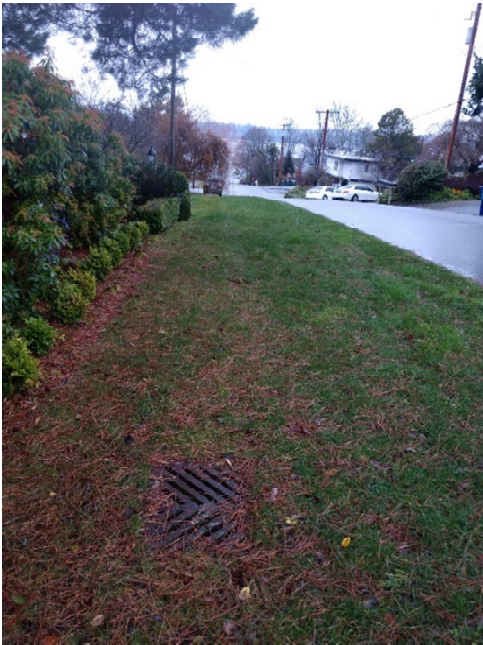
Photo N4 – Facing west along SE 28 th St approximately 130 feet west of Photo N3. Runoff is conveyed via this catch basin on the south side of the street toward Lake Washington.
