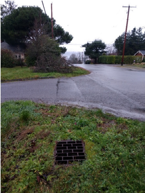
Photo N3 – Facing west along SE 28 th St approximately 145 feet west of Photo N2. This catch basin is located adjacent to the driveway into the back parking lot on the western portion of the property. Runoff continues to sheet flow northwest towards the conveyance system on the south side of the street.
