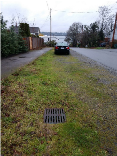
Photo N6 – Facing west along SE 28 th St approximately 150 feet west of Photo N5. Runoff is conveyed via this catch basin on the south side of the street toward Lake Washington.
