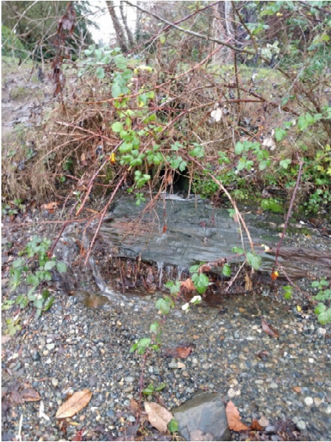
Photo S14 – Facing east looking directly at the outfall to Lake Washington.
