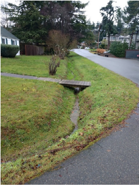
Photo S7 – Facing east along the north side of SE 30 th St approximately 210 feet west of Photo S6 at the northeast corner of the intersection of SE 30 th St and 61 st Ave SE. Runoff is conveyed west toward Lake Washington.
